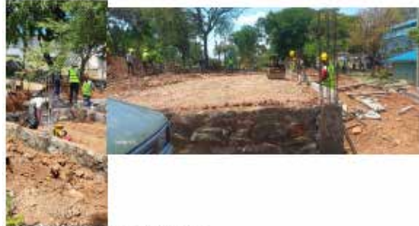
LEVELING AND COMPACTION
