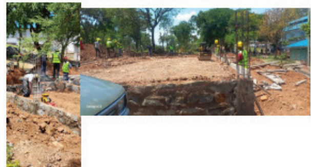
LEVELING AND COMPACTION
