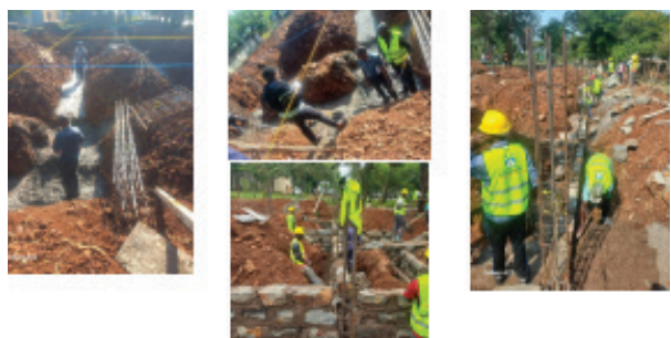
STRIP FOUNDATION & FOUNDATION WALLING
